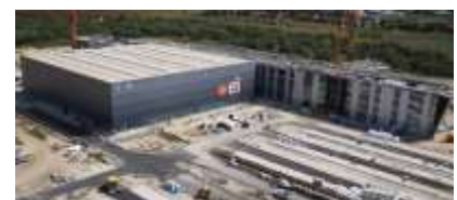
Construction Site Video
