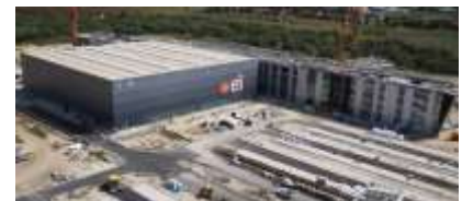
Construction Site Video
