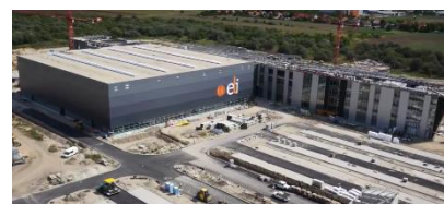
Construction Site Video
