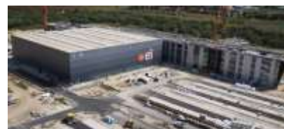
Construction Site Video
